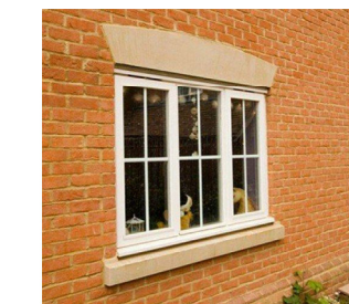
New cast stone lintels and cills
