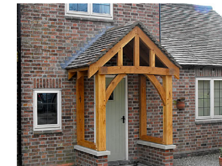
New Porch to look like this
